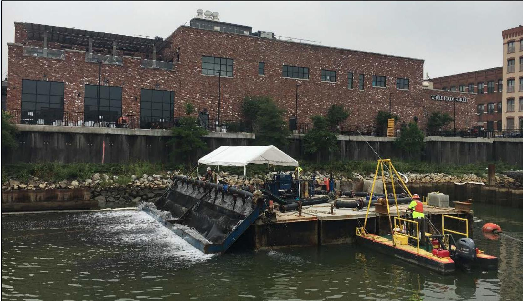
A minimum of 4 inches of GAC and sand was designed to be placed and on average a total of 7 inches were placed within the hydraulic demonstration footprint. Hydraulic capping was selected as the preferred method and used to place the treatment layers in the full scale Pilot Area. The sand-based isolation and filter layer was also placed via hydraulic capping.
