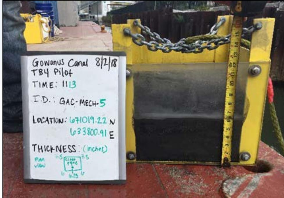
**Catch Pans** were deployed prior to placement of each layer and retrieved after confirmation coring in order to verify the thickness of the placed cap.
